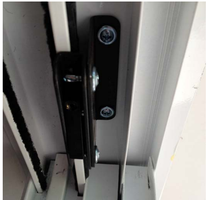
View looking up at mounting bracket and gravity latch mounted on underside of door frame
