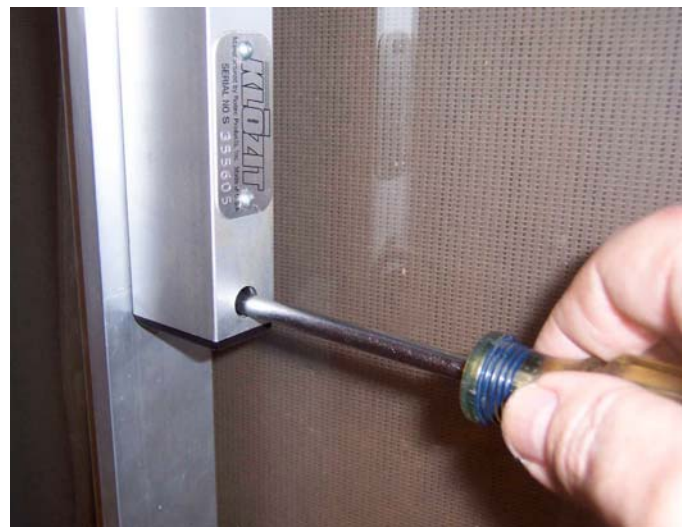
Attaching bottom mounting screw
