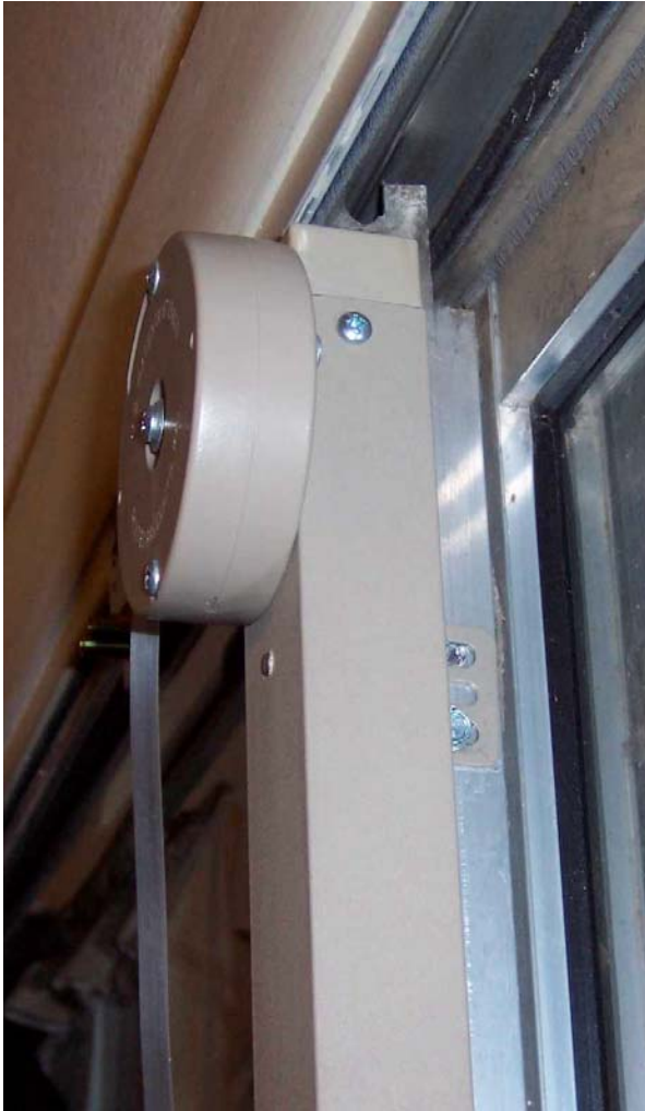
View of top of strap type closer showing upper spool and upper mounting bracket
