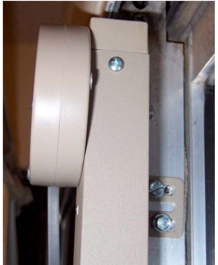
Close-up of strap type closer showing upper mounting bracket and clearance to door frame
