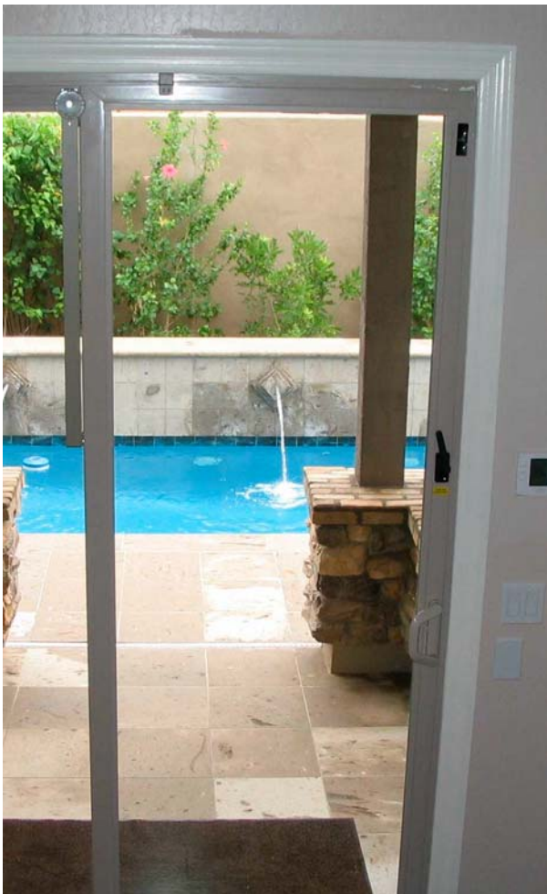
Strap type closer mounted on right-to-left opening door. KLOZIT door latch mounted above existing door handle
