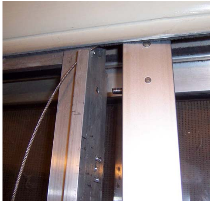
Cable closer top view showing rollpin being inserted into hole
