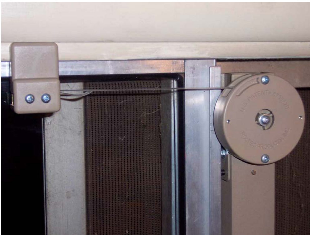
Close-up of strap type closer showing tape spool and tape anchor with cover attached
