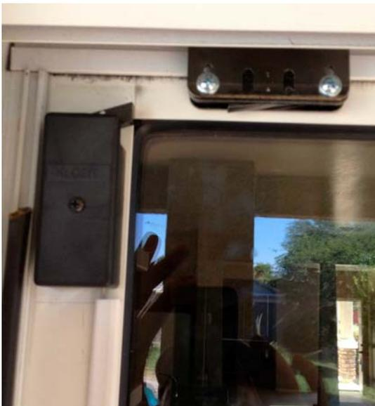
Latch body (left) with cable coming from below, concealed by white plastic cable cover. Latch striker in locked position
