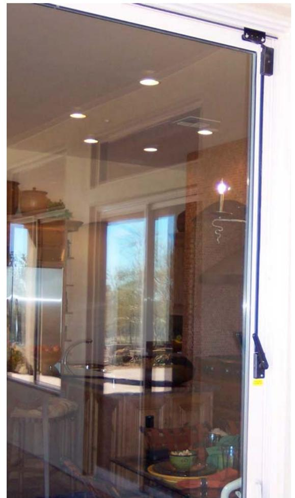
**Exterior view of door latch system with Latch handle, plastic cable cover, latch body and gravity latch bracket visible.**
